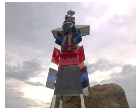
Inspecting and servicing Rua Dika rock light
